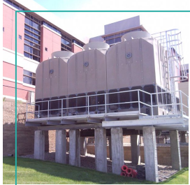
Evaporative Cooling Towers
