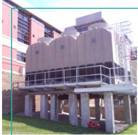
Evaporative Cooling Towers
